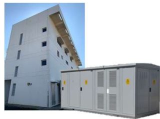
PSA Smart Grid Deployment & Electrical Infrastructure
